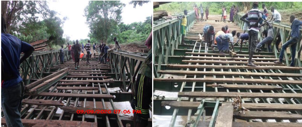
Figure 6: Returning and replacing the broken pieces of timbers on the bridge
