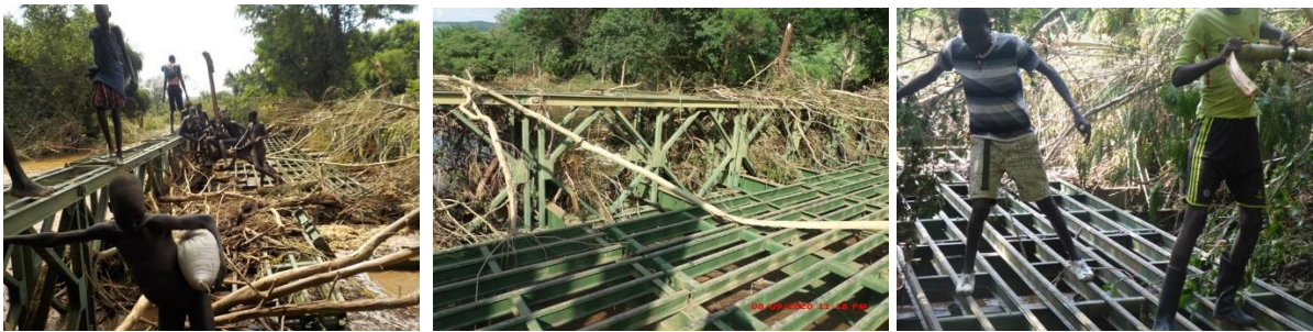
Figure 4: Damage caused by the flood on the motor bridge and volunteers cleaning the debris
