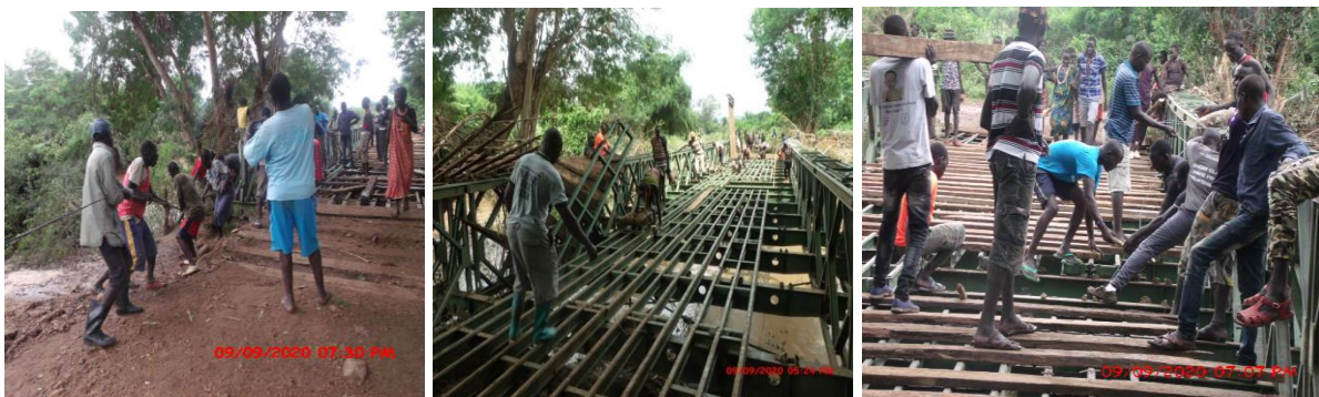
Figure 5: Recovering metals and timbers from the water on to the bridge.
