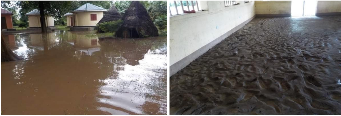
Figure 8: The whole compound was flooded and in all the houses where deposition of sand.
