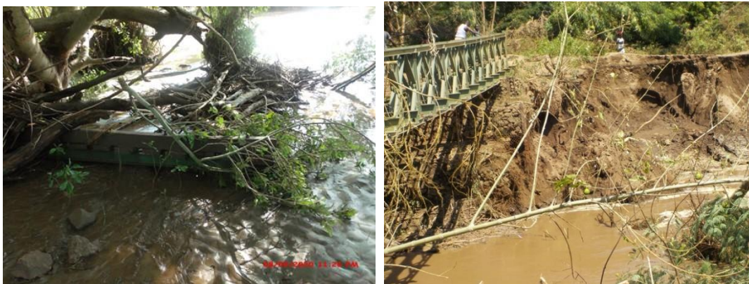
Figure 7: Severe erosion caused by the flood at the foot of the motor bridge
